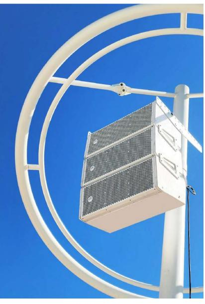
The audio for the main dance floor is primarily delivered through twenty eight WR-320-DXW line array systems, reinforced by six SARA-SUB-W subwoofers and WR-218S-DXW subwoofers dedicated to the dance floor. Several ARTEC series systems provide the necessary additional fill.
